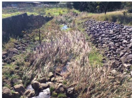
Image 63 – Part of Creek restoration work in Bonnyrigg District Park
